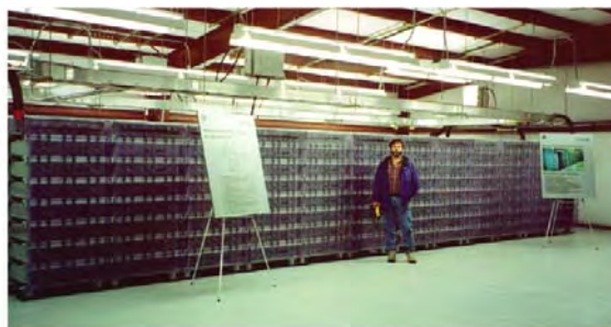
Figure 4-7 1-MW/1.5-MWh Lead-Acid System at Metlakalta, Alaska
