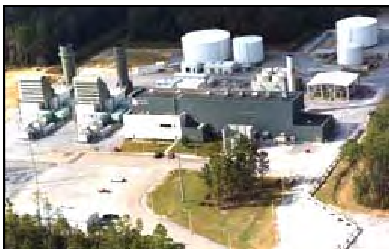
Figure ES-2 Underground CAES Plant, Alabama
