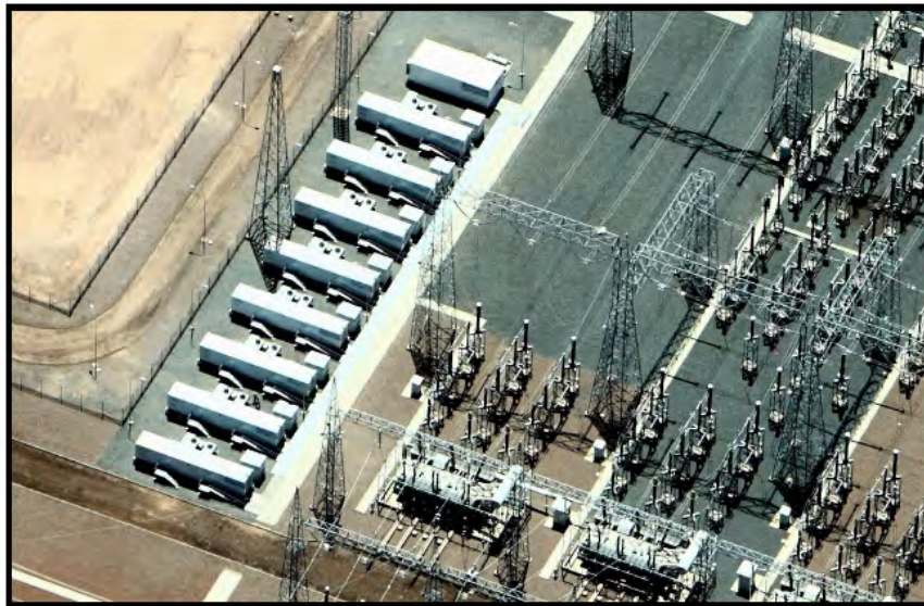
Figure ES-7 Commercial operation of a 12-MW frequency regulation and spinning reserve project at AES Gener's Los Andes substation in the Atacama Desert, Chile. The system uses A123 Systems' Li-ion Hybrid Ancillary Power Units (Hybrid-APUs™).
